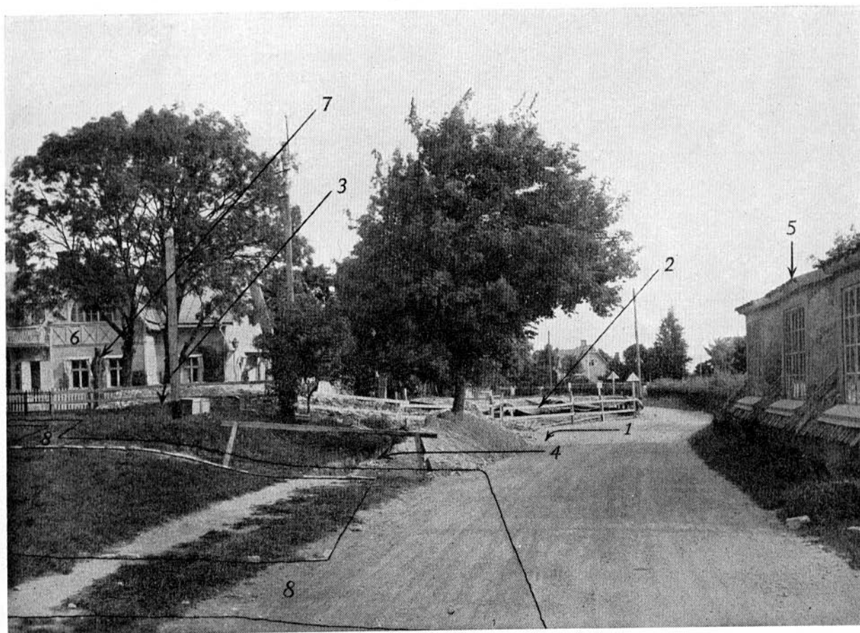
Fig. 40. Excavation area at Korsbetningen. For explanation of figures, see fig. 39.
