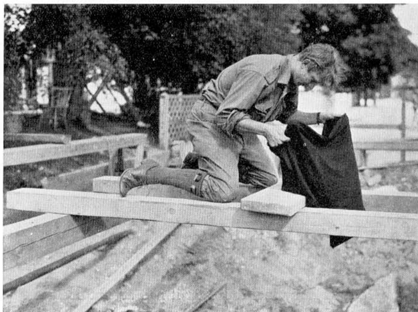
Fig. 57. Photographing from roof-beams.
